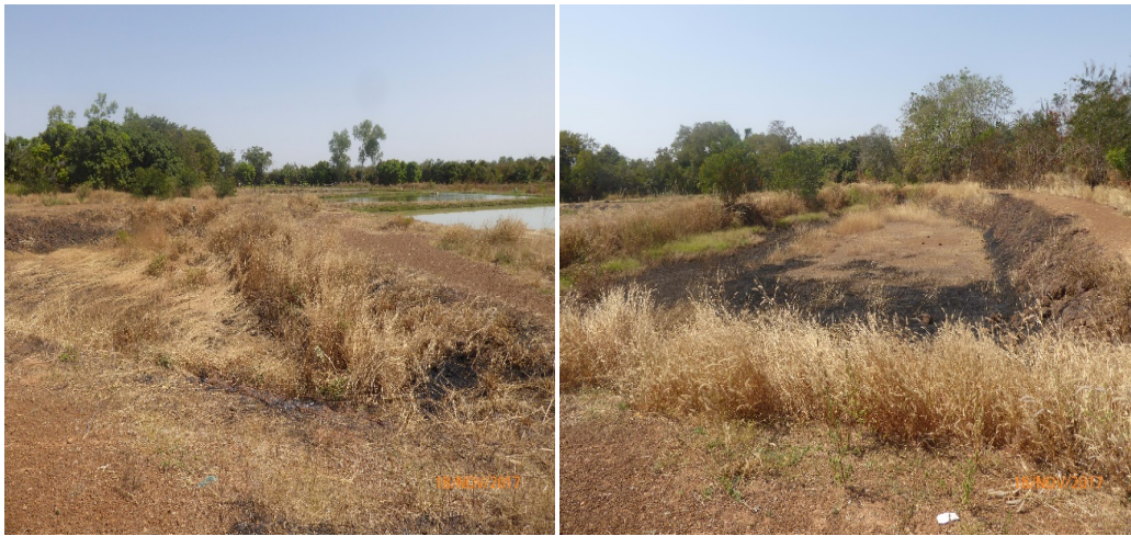
Figure 54: Bazèga Aquaculture Station: Ponds unable to be filled with water by gravity (Source: R. Ouédraogo)
