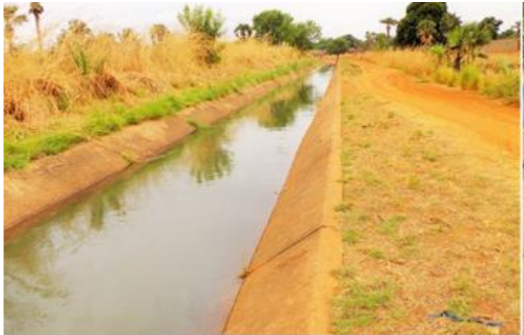
Figure 10: example of channelisation in Burkina Faso (Source: Idrissa Kaboré)
