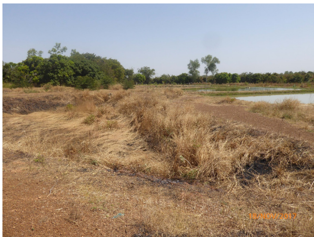
Figure 37: In the governmental aquaculture farm of Bazèga, some fish ponds cannot be filled with water (Source: R. Ouédraogo)
