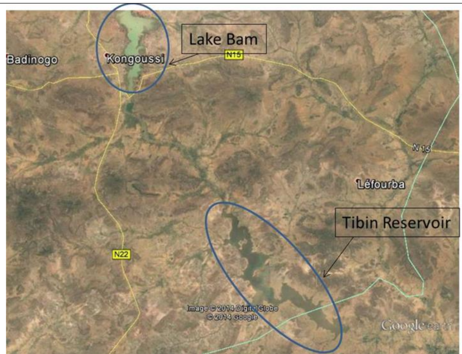
Fig 1: The new reservoir of Tibin is located 20 km downstream Bam Lake (From Google Earth, 16 April 2014)
